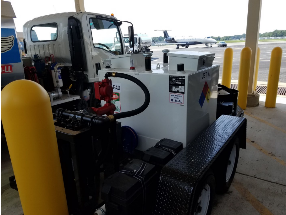
200-Gallon (100-Gallon/Each Tank) Jet A/Aviation Gasoline Mobile Fuel Sump Cart (FS-2M) Parked by Tank Trucks Between Terminal and Self-Fueling Pumps
