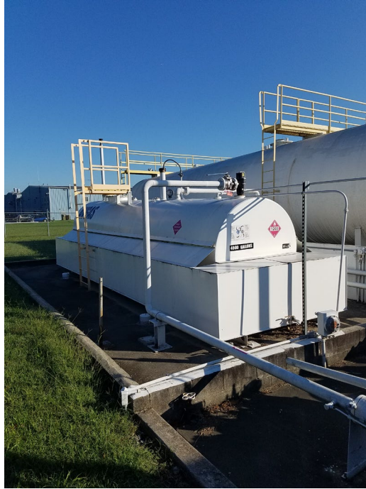
4,000-Gallon Aviation Gasoline Tank (FF-13A) At Fuel Farm – West Containment Area
