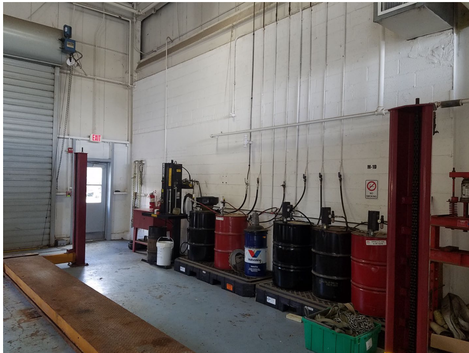
55-Gallon Drums of Motor Oil, Transmission Fluid, and Hydraulic Fluid for Vehicle and Equipment Use (M-1D) Inside Maintenance and Auto Shop (Building 9) – North Side
